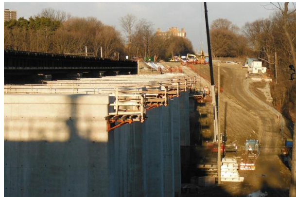
The Georgetown South Project
