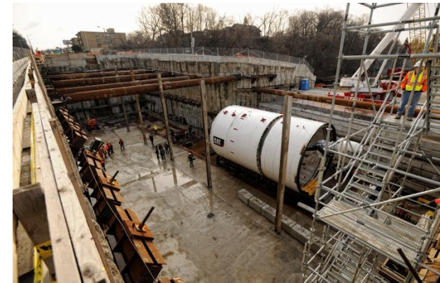
Toronto Light Rail Transit including Eglinton Crosstown
