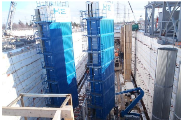
Toronto–York Spadina Subway Extension
