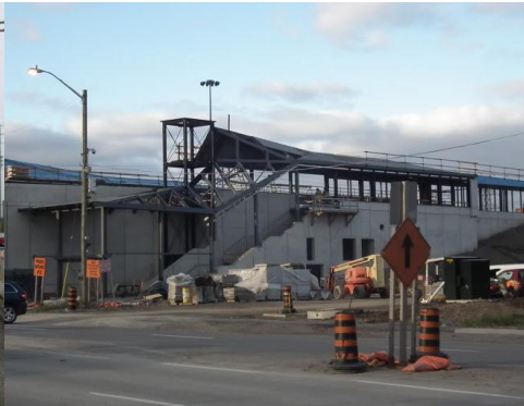
Mississauga Bus Rapid Transit
